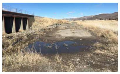
The golf cart paths are surfaced with asphalt; in some locations, there is periodic inundation with water resulting in sedimentation (left). Veteran's Parkway construction removed some paths, leaving "deadends" that could be removed and revegetated (right).
