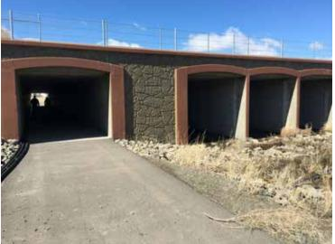
The tunnel below Veteran's Parkway as seen looking west (left). A series of tunnels at the southern end of the site convey water, with one tunnel providing access via a paved pathway (right).
